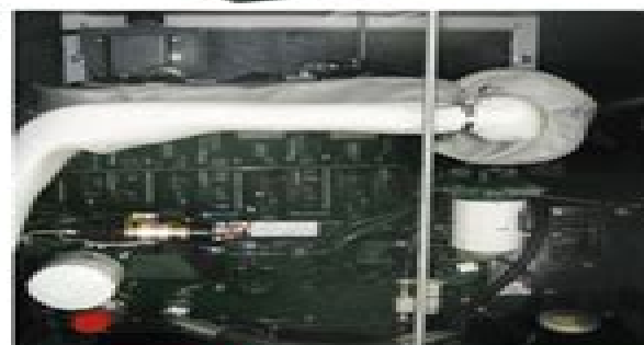
Detail of interior
